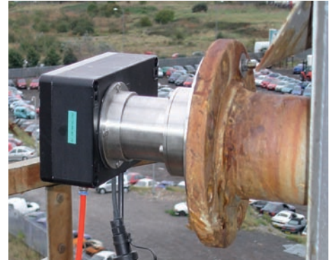
Gas Fired Boiler monitored by Pro-Scatter Technology
